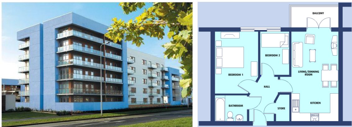
Figure 3. Image and typical floor plan of one of the case study apartment buildings © Coastal Housing Group Ltd.
