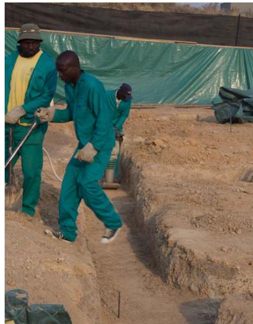
Figure 5 Polymer stabilised layer chopped down to level
